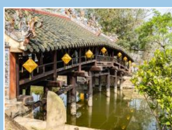
Than Toan Bridge
