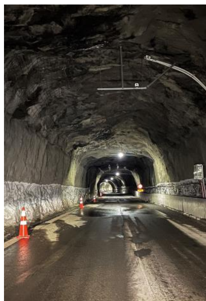
Homer tunnel – Fiordland
